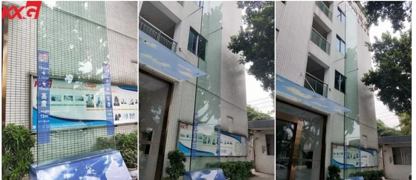
19 mm +2.28 mm SGP +19 mm SGP SGP 19.19.3 2 19 mm 2.28 mm SGP interlayer 19 55 19 55 19 55 19 55 19 55
