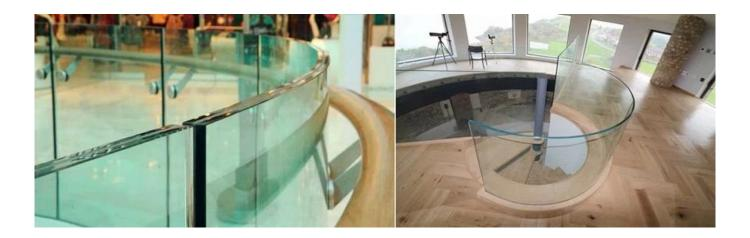
21.52mm low iron curved toughened laminated glass railing
