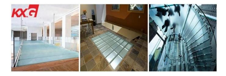
The matte non-slip glass floor is made of frosted glass surface, and the glass surface is very rough to achieve anti-slip effect. This type of floor glass has a good anti-slip effect, but is not easy to clean, so it is less preferred by the market.
